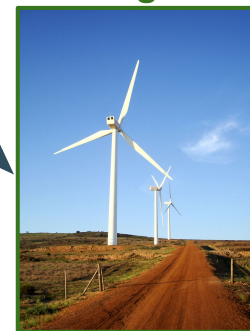
Wind turbine 2 target
